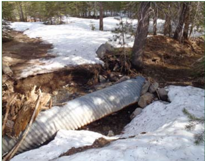
This culvert will be replaced with a rock-hardened low water crossing.
