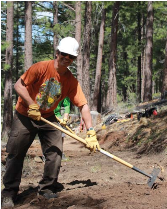
A volunteer uses a McLeod to build a new trail segment at Waddle Ranch Preserve.
